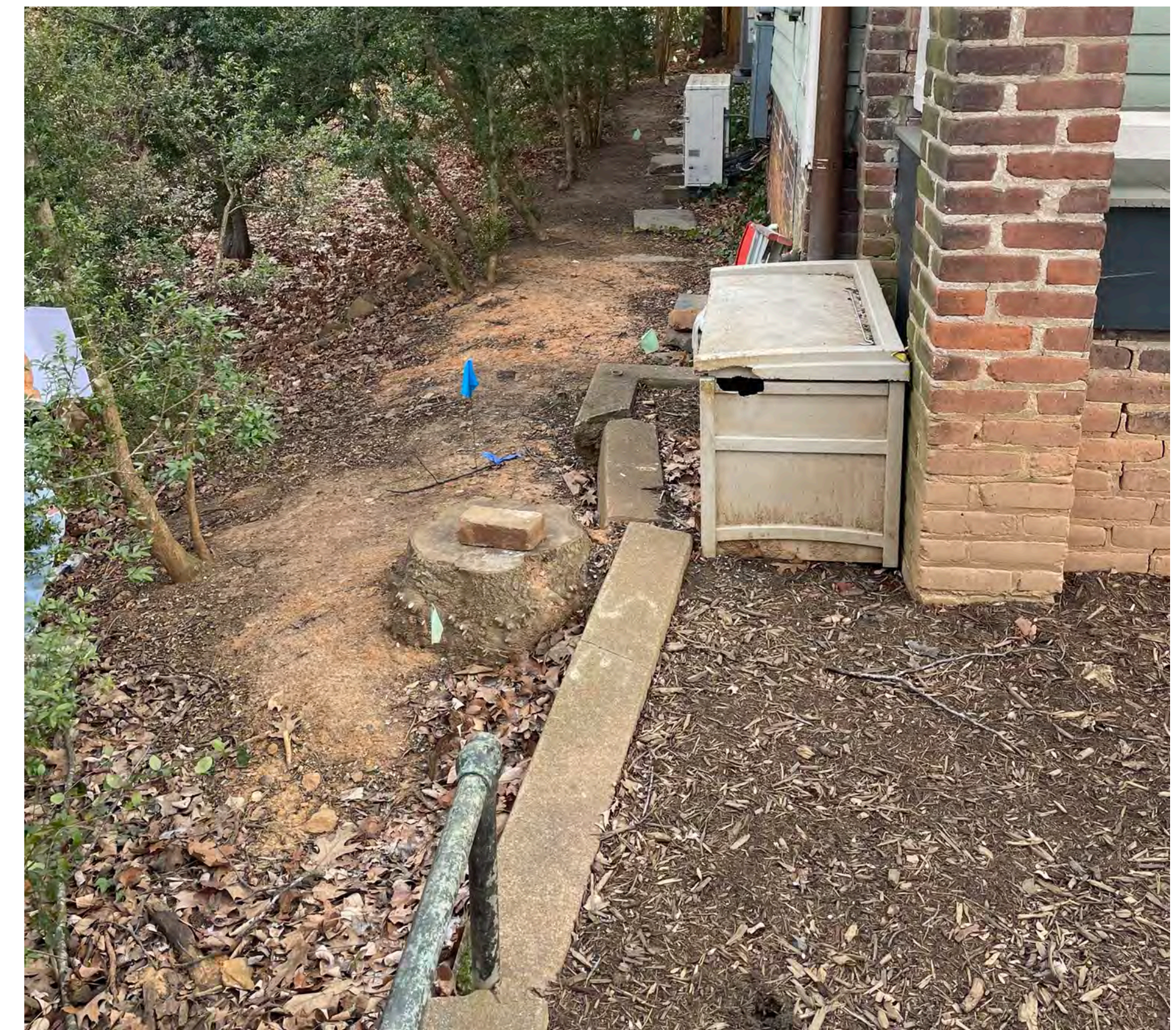
BROKEN CONCRETE WALL FOR REMOVAL. PATCH & REPAIR REMAINING RETAINING WALL.
