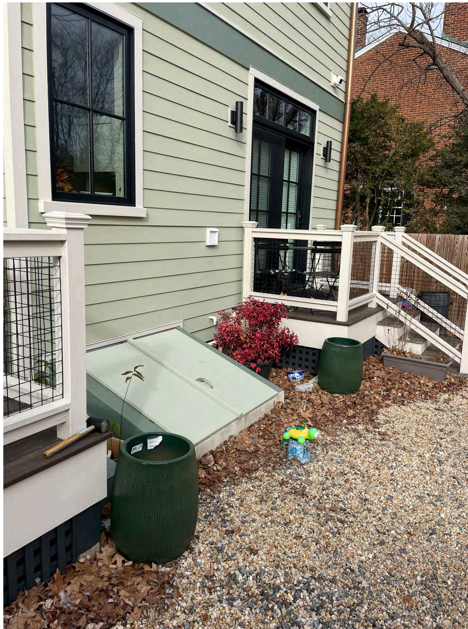
EXISTING REAR PORCHES & GRAVEL TERRACE.
