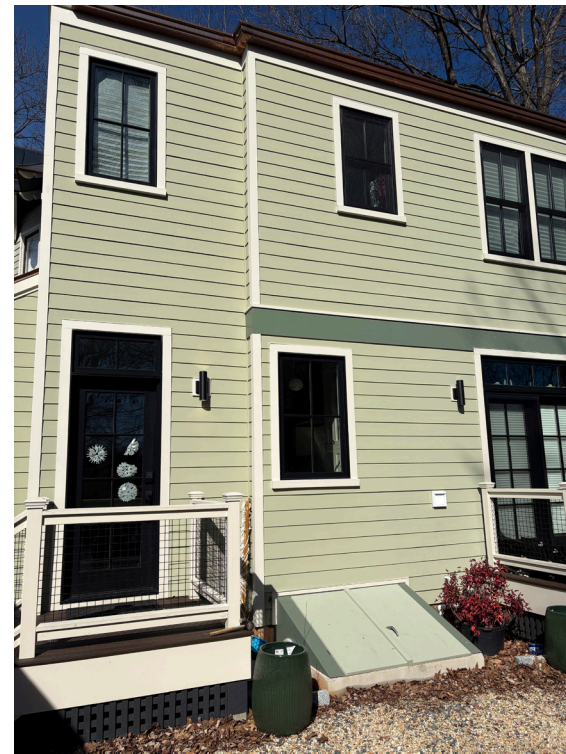
Existing house, east facade
