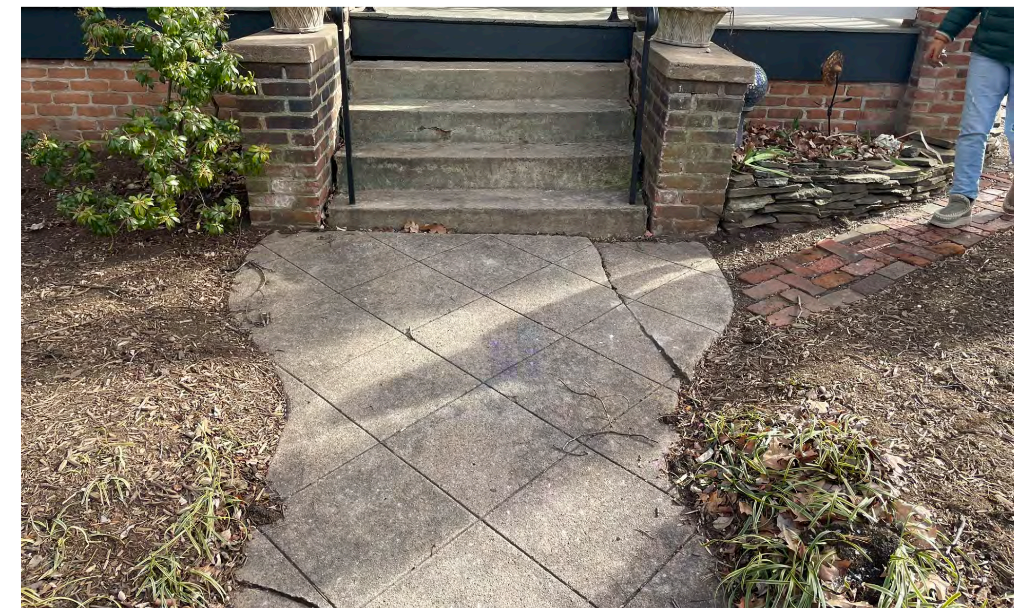
CONCRETE STAIRS & PATH FOR REMOVAL.
