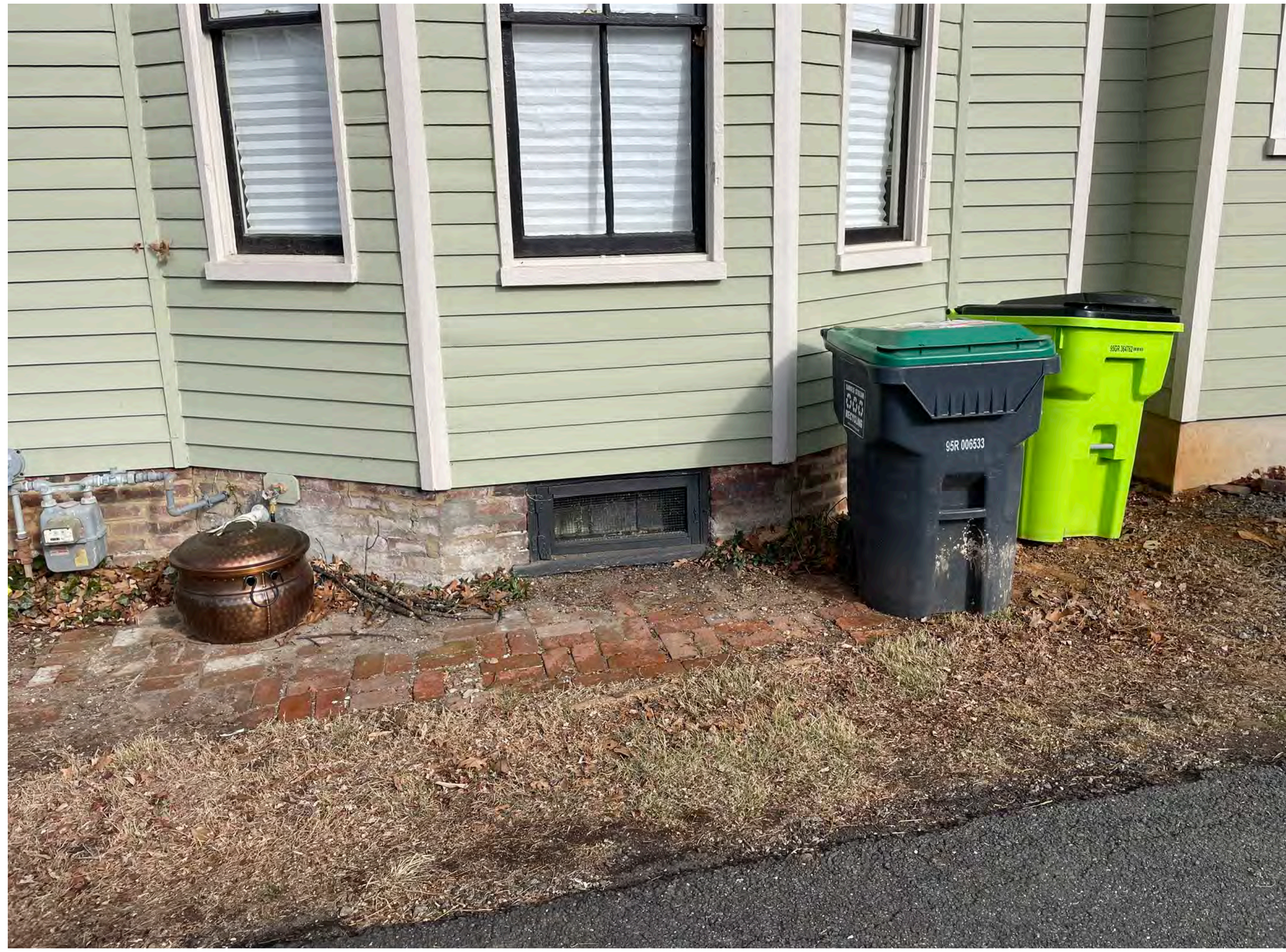
EXISTING TRASH STORAGE & SIDE ENTRY AT EASEMENT.
