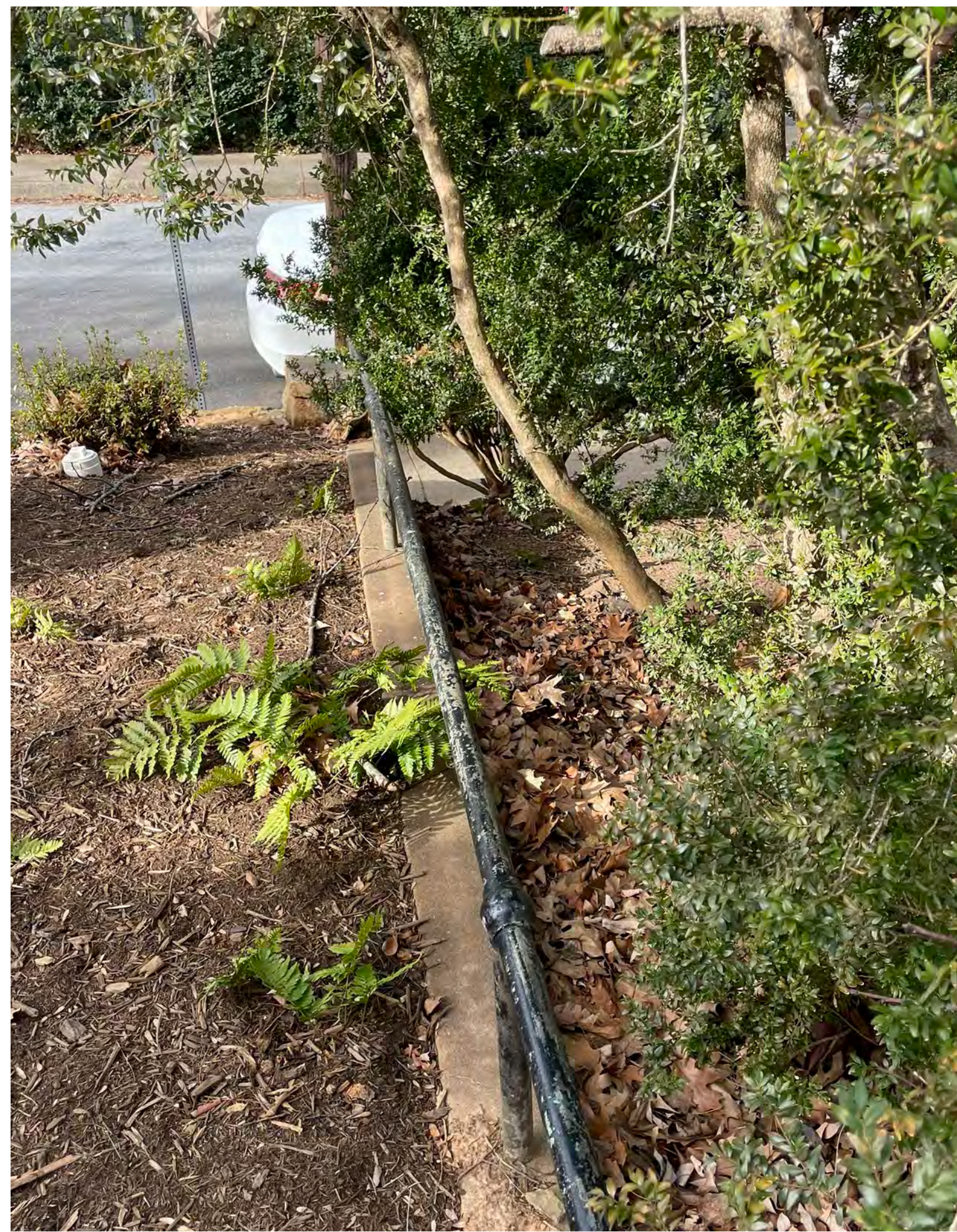
RETAINING WALL & BOXWOODS TO REMAIN.
