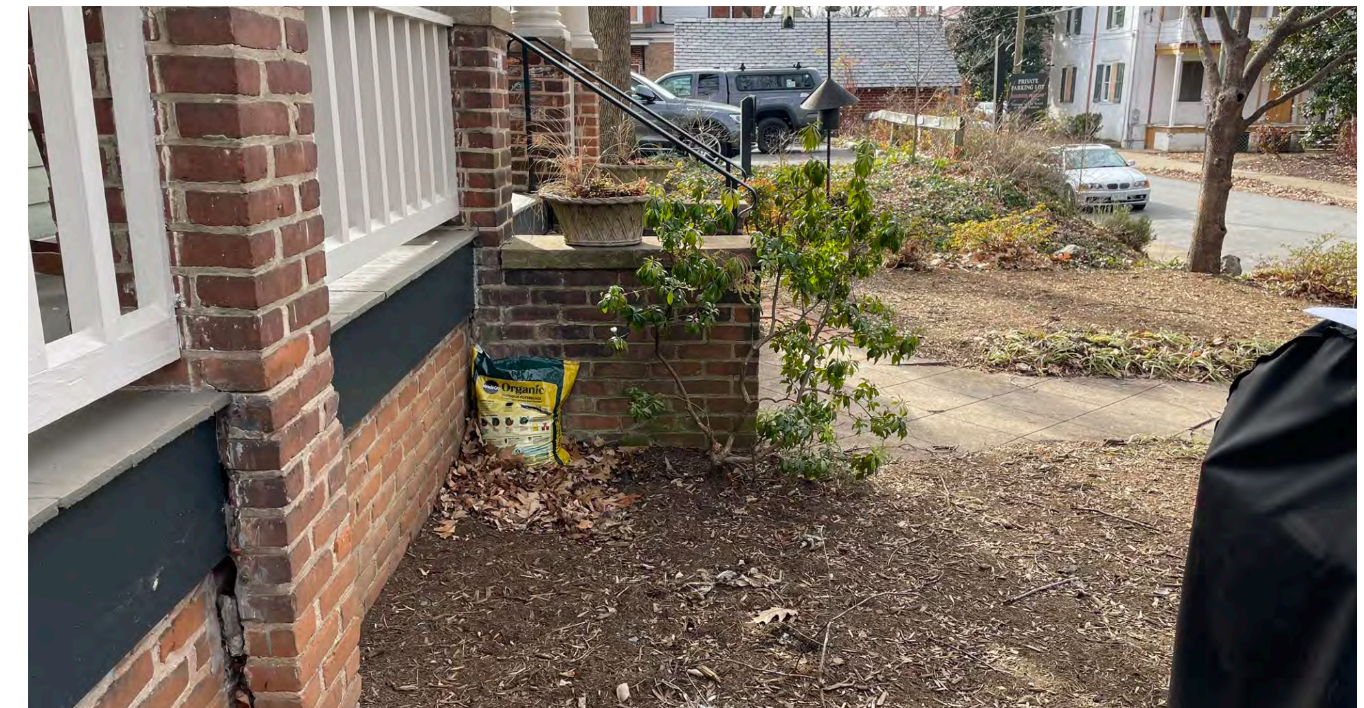
EXISTING FRONT STAIR CHEEK WALLS & PATH.
